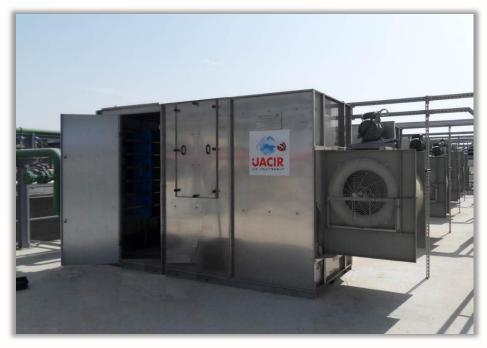
Range: water flow rates from 6 to 190 m3/h Power from 20 to 2 000 kW
