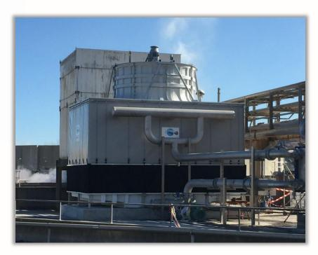
Water flow rate: from 250 to 10 000 m3/h Power: 1 450kW to 58 000kW
