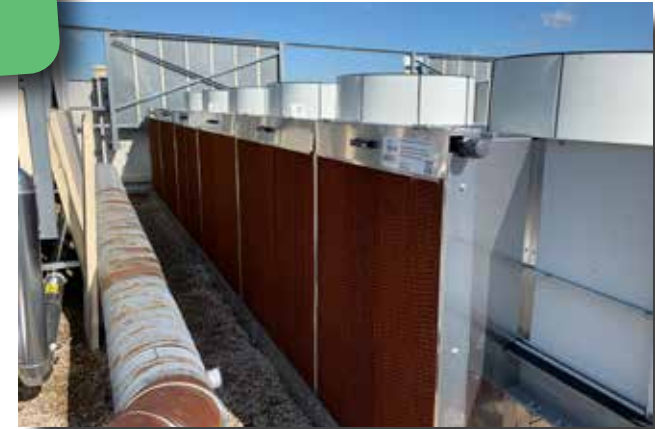
Optimised performance BoostCooler ® 513 kW - 51/45°C @ 41°C Ext.
