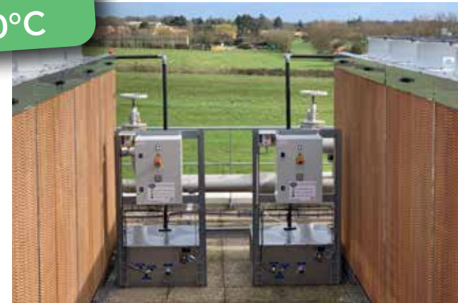
Optimised performance BoostCooler ® 725 kW - 35/30°C @ 35°C Ext.
