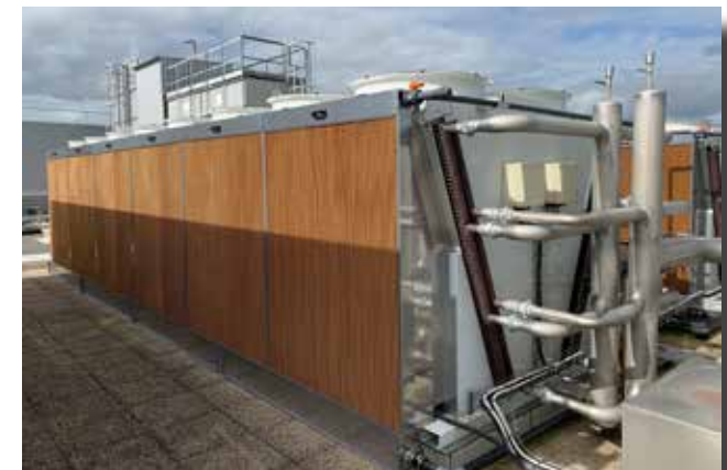
Optimised performance BoostCooler ® 725 kW - 35/30°C @ 35°C Ext.
