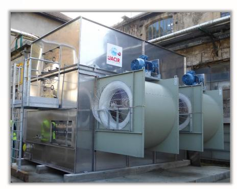
Water flow range from 74 to 766m3/h Capacity: 1100 to 3300kW
