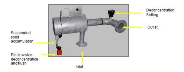
In addition to the original fouling resistance of the exchanger (high water velocity), this equipment is designed to retain suspended solids in the water. Those are nourishment enhancing bacteriological growth. Its characteristics are:
