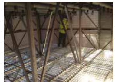
Slatted floor under the infill for easier and faster maintenance
